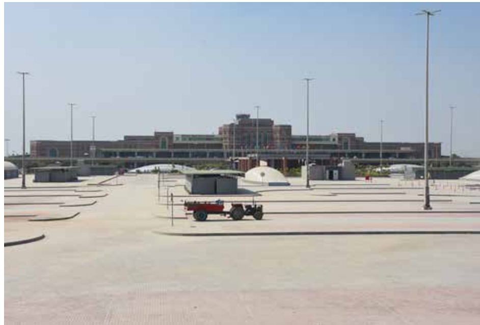
Allama Iqbal International Airport, Parking expansion, Lahore
